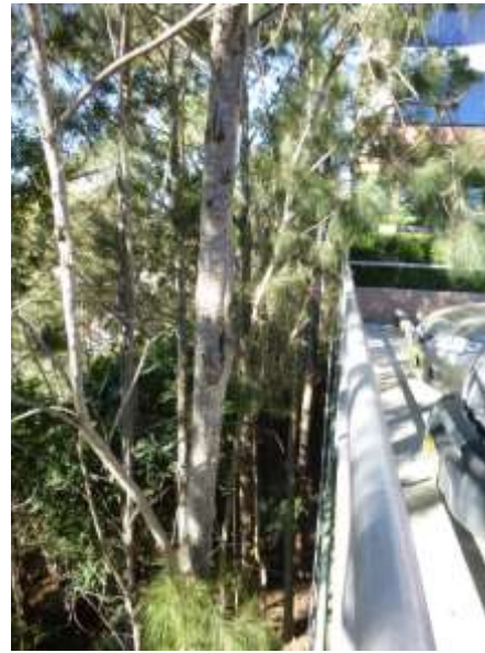
PICTURE 2 – STEEP DROP IN GROUND LEVEL AT NORTHWESTERN BOUNDARY OF 18-20 ORION
